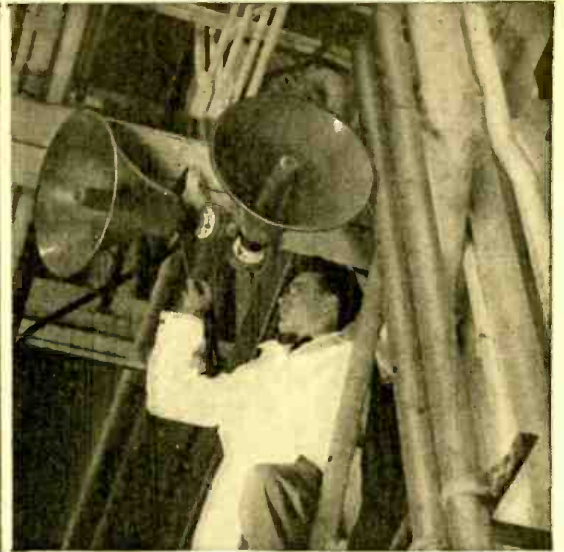
Above—Two of the Atlas Sound DR-42 Dynamic Reflex Projectors installed in the Pratt & Whitney Aircraft engine assembly building. There are 3 speakers in the cluster, one being hidden by the column. Left—Three 75-watt power stages mounted in rack, together with two-position mixer. Switching permits progressive paging by groups of seven speakers to each power stage. The whole system is controlled from one point, where a "grip-to-talk" microphone is used.
