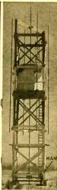
Photo above shows operator at airport checking direction of plane transmitting regular communication signal. The receiver employs an Azimuth-indicating device, operating in the 2 to 7 megacycle band. Right—Note size of man and the dipole antennas. Below—Diagram of receiver and arrangement of dipole antennas.
