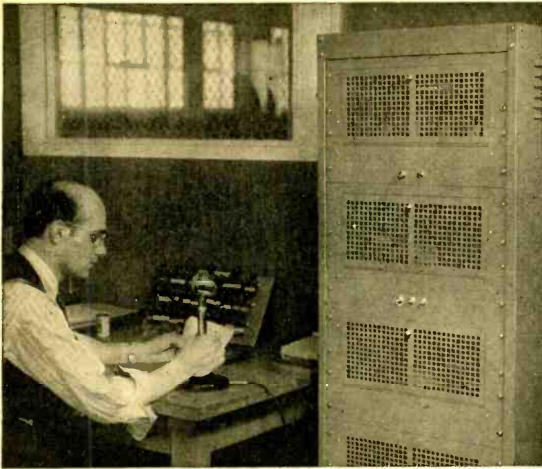
Above—Two of the Atlas Sound DR-42 Dynamic Reflex Projectors installed in the Pratt & Whitney Aircraft engine assembly building. There are 3 speakers in the cluster, one being hidden by the column. Left—Three 75-watt power stages mounted in rack, together with two-position mixer. Switching permits progressive paging by groups of seven speakers to each power stage. The whole system is controlled from one point, where a "grip-to-talk" microphone is used.
